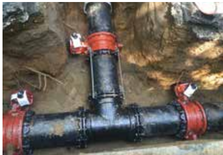
New 16-inch water main
